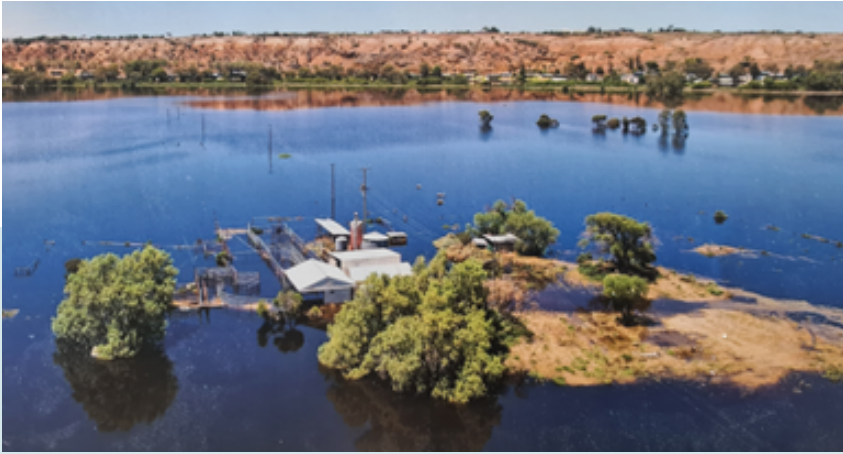
The effects of the 2022 flood Photo supplied by Jenni Llewellyn
